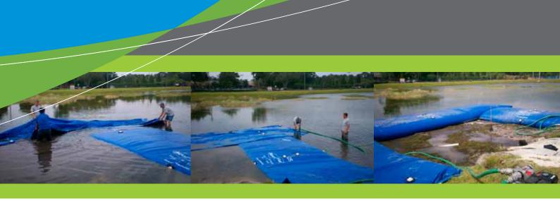
Aqua Barriers are folded and rolled onto standard pallets enabling easy transportation and site handling. Once on site the pipe loops at each end of the Aqua Barrier enable the Aqua Barrier to be moved around site and into the water. The filling process is fast and straightforward with simple connections between the Aqua Barrier and on-site pumps.
