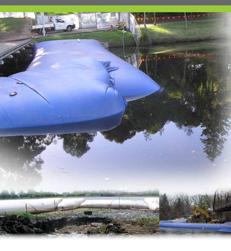
Aqua Barriers are also be used in flood control projects, taking advantage of their speed of deployment. They have been used in Australia by the SES as well as in Thailand, during their extensive recent flooding. Once the flood has receded, the Aqua Barriers are deflated, rolled, palletized and stored for re-use.
