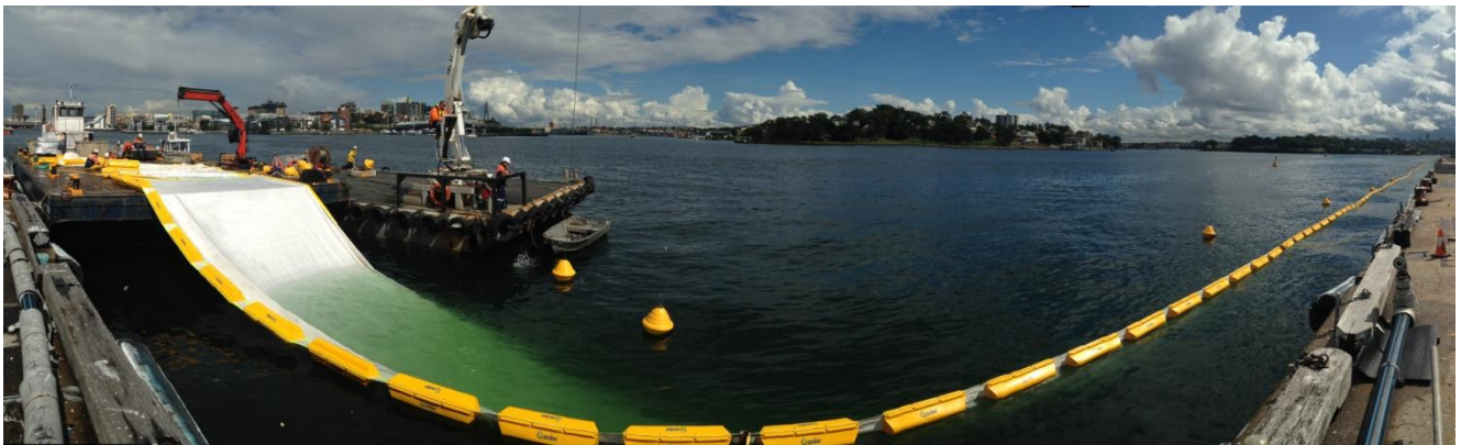
Deployment at Barangaroo, Sydney Harbour, NSW Custom Heavy Duty Silt Curtain
