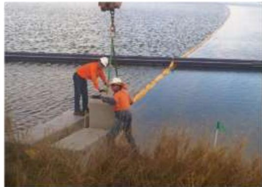
The skirt is gathered and pre-tied to the baffle's floats, then packed as a concertina then packed for easy unloading and deployment. Multiple sections of GeoPro Floating Baffle will be joined together and packed onto the pallet or crate. Where the total length of baffle system requires multiple pallets to ship, individual sections (of multiple panels) will need to be joined at the time of deployment to create the complete system.
