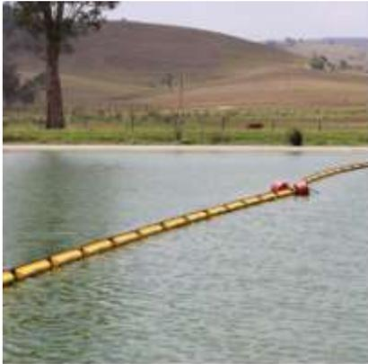
GeoPro Floating helps to improve the operation efficiency of a waste water treatment system. GeoPro Floating Baffles are used in sewage treatment plants, industrial waste water treatment plants or other treatment processes related to mining or the oil and gas sectors.
