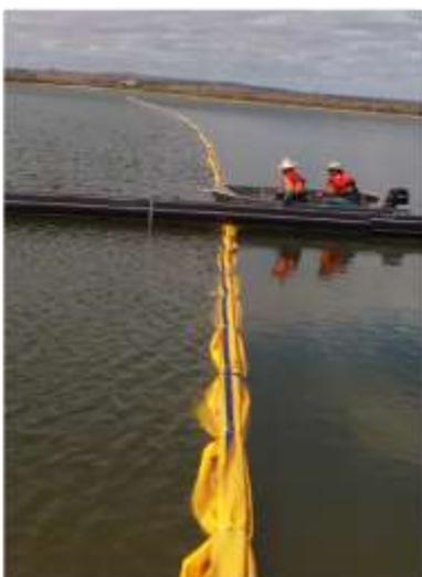
As the baffle is being deployed, it is floated across the lagoon to its anchoring destination on the opposite embankment. This can be accomplished with the aid of a small boat and a line, or a line can be run from the baffle's far end connection across the lagoon to the opposite shore to pull the baffle across.
